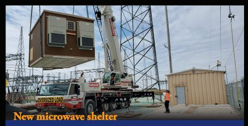
**Above** Crews place a new microwave shelter at a MidAmerican Energy site, moving Corn Belt Power closer to finishing its southwest microwave loop project. The project will enhance reliability of the cooperative's communication system.
